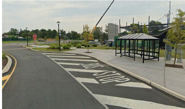
Bus stop with a shelter and lighting for LANTA serving commercial developments in Lower Macungie Township, Lehigh County
